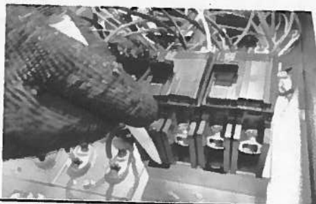
Pull the lock of the bottom breaker and remove the breaker from the sheet metal base.
